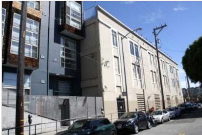
Photograph 147. 466 Townsend Street, secondary elevation.
