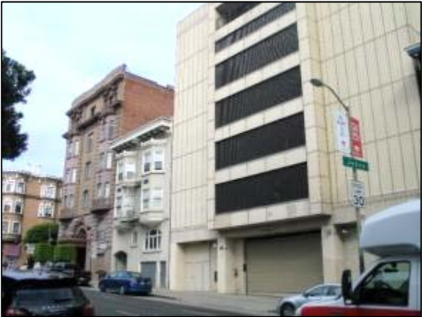
Photograph 92. Mid-block Pine Street, facing northwest.
