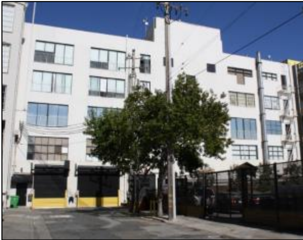
Photograph 125. 58–60 Federal Street (ES-30).
